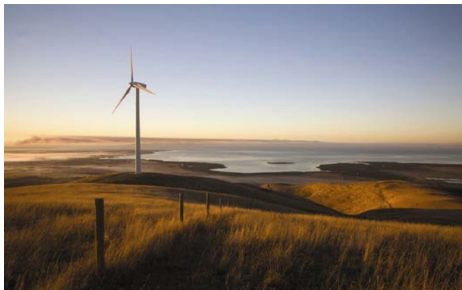
Toora, Vic - 21MW
