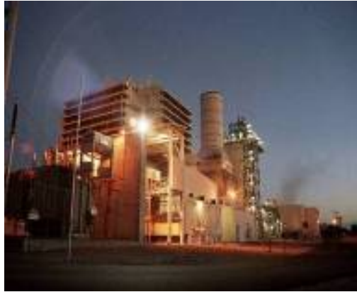
Townsville Power Station – 230MW
