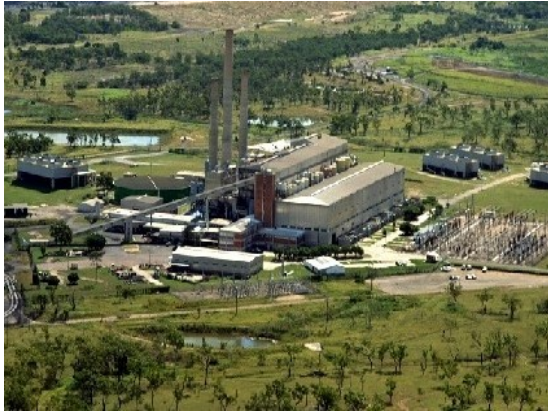
Collinsville Power Station - 180MW
